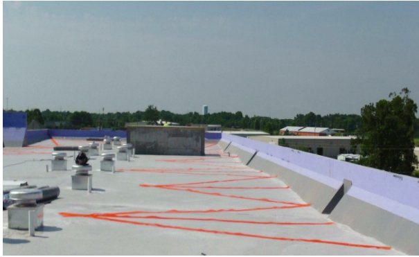
Distribution Strips Connect the Roof Perimeter to the VacuSeal™ roof vents
