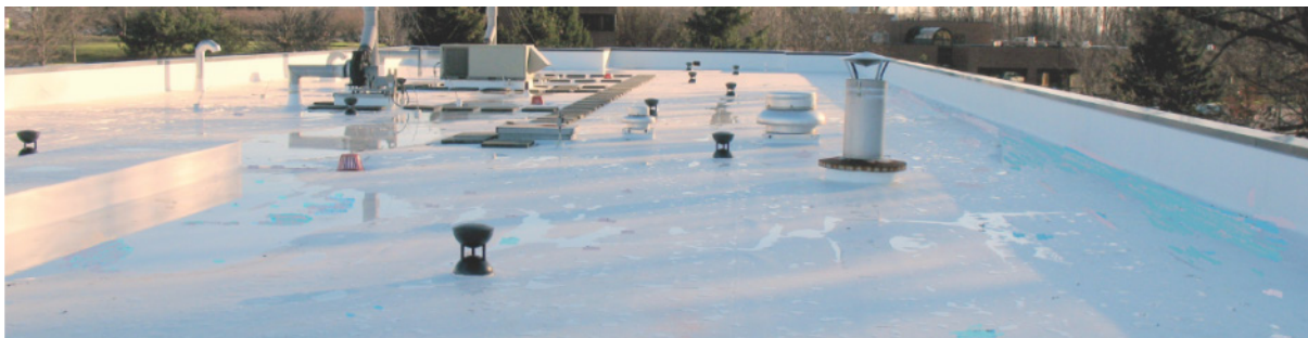
Position of VacuSeal™ roof vents are Staggered to Accommodate Variations in Wind Speed on a Completed Roof Application
